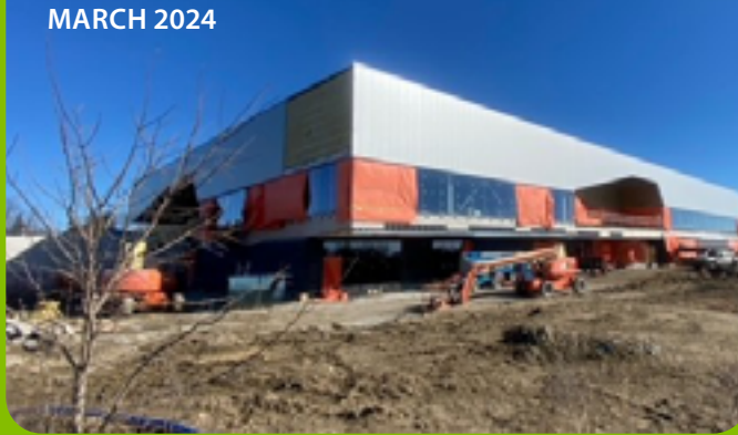
CARRVILLE LIBRARY CONSTRUCTION AS OF MARCH 2024
